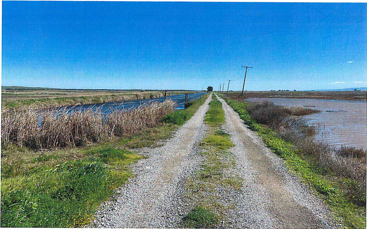
Photos of Reclamation District #2129 Levee Road and Water Supply Ditch
