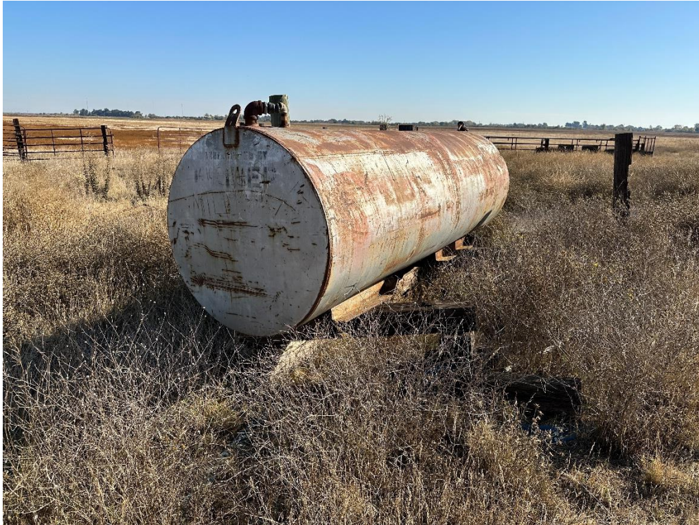
Photo No. 9 Approximate 1,000-gallon water aboveground storage tank along western side of the corral
