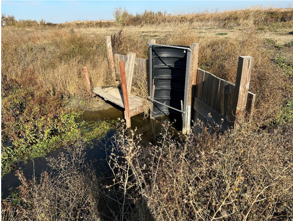
Photo No. 17 Water flow control gate in northeastern portion of the site (open to actively flood northeastern portion of the site)
