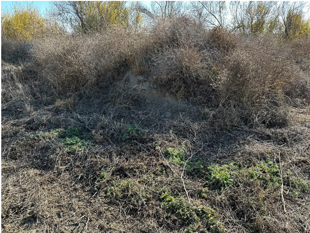
Photo No. 16 Soil stockpiles adjacent to the southwest of the pole-mounted transformer
