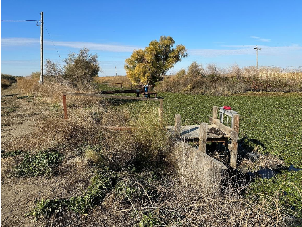
Photo No. 15 Water flow control gate in irrigation canal (which feeds water to the northern portion of the site)
