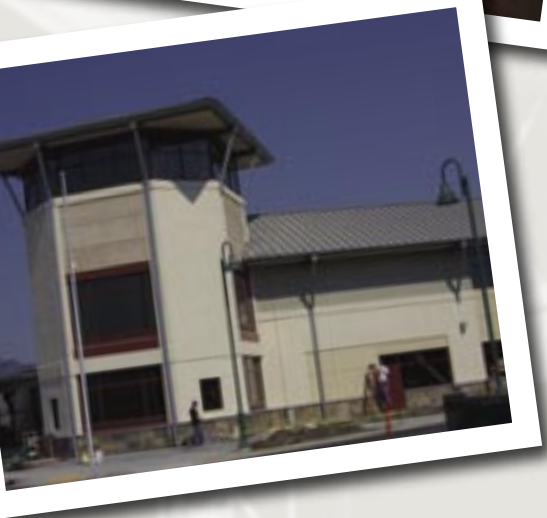
Top to bottom: Dedication of future William J. Carroll Government Center by Supervisors Duane K. Kromm, John M. Vasquez, Michael J. Reagan, Vacaville Mayor Len Augustine and Council members Steve Hardy and Steve Wilkins; Nut Tree Airport improvements; County implements new voting machine; new Cordelia Library.
