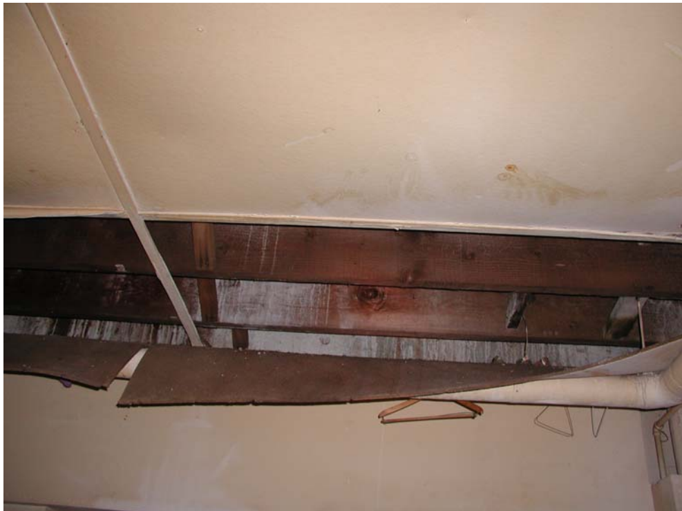
First floor joists (seen from basement level) (March 2008)
