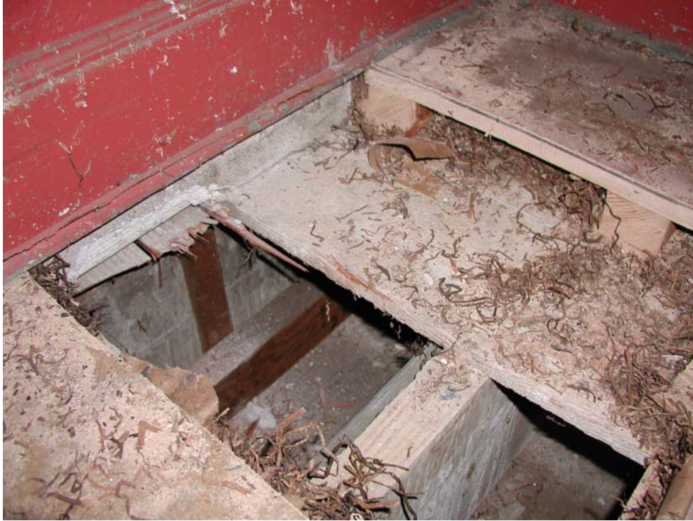
Exposed second floor framing (auditorium)
