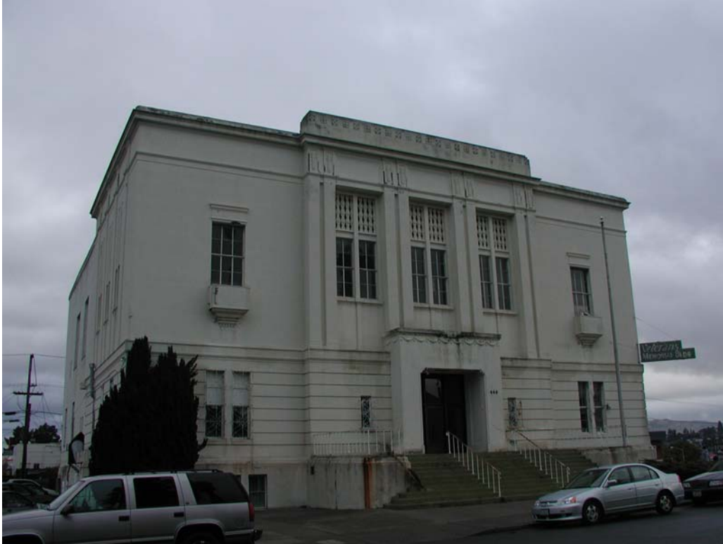
Front Entrance - South Elevation (March 2008)
