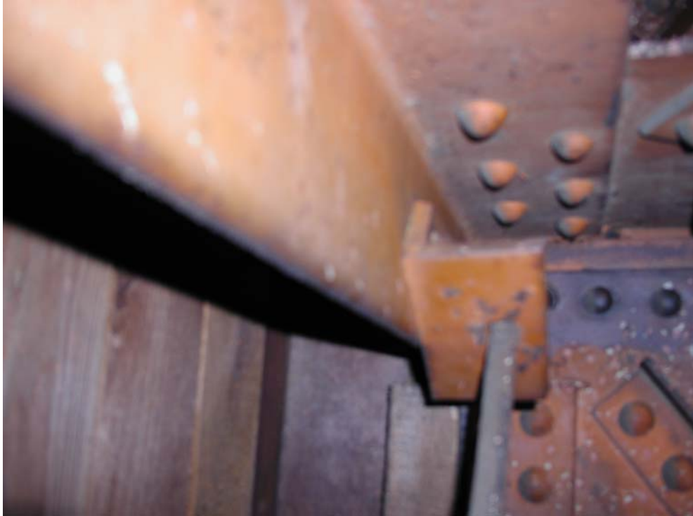
Riveted connections at roof trusses
