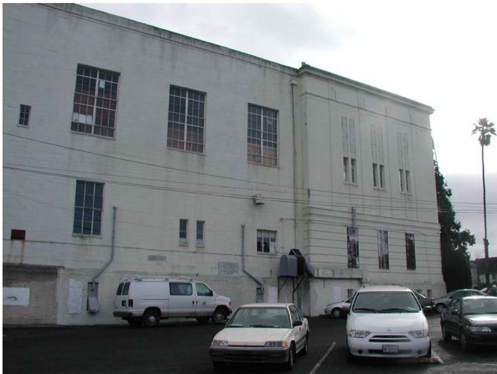
West Elevation at parking lot (March 2008)
