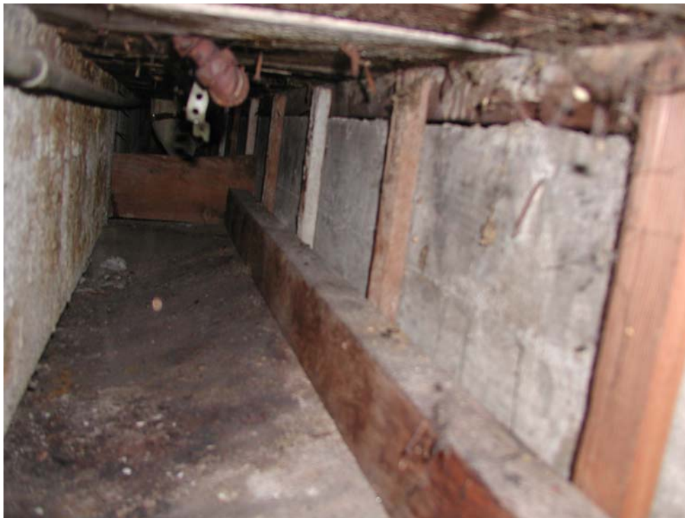
Second floor framing from access hole (March 2008)
