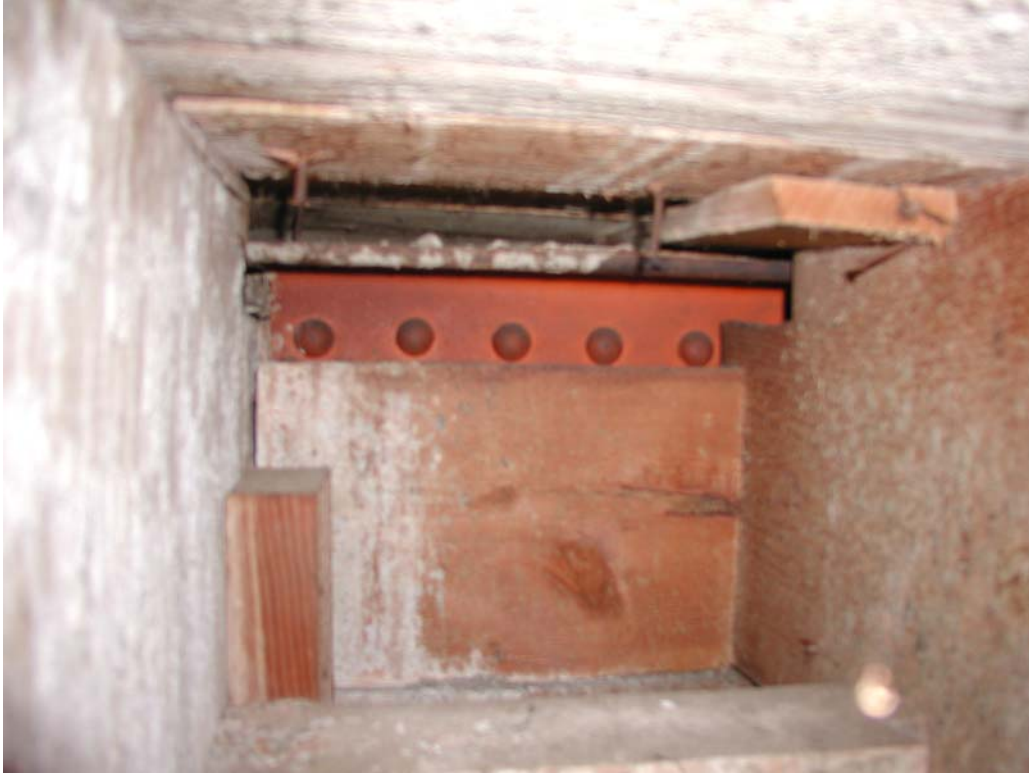
Second floor framing looking toward beam to pilaster at access hole
