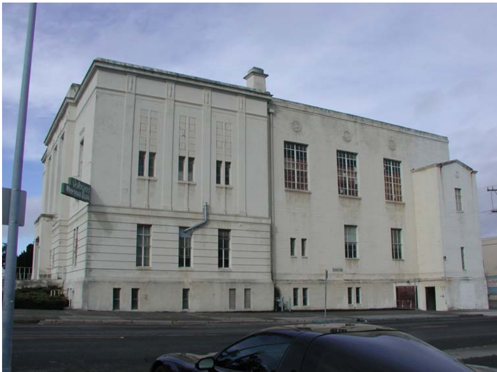
East Elevation (March 2008)
