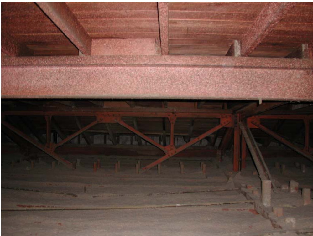
Roof trusses, rafters and straight sheathing (March 2008)
