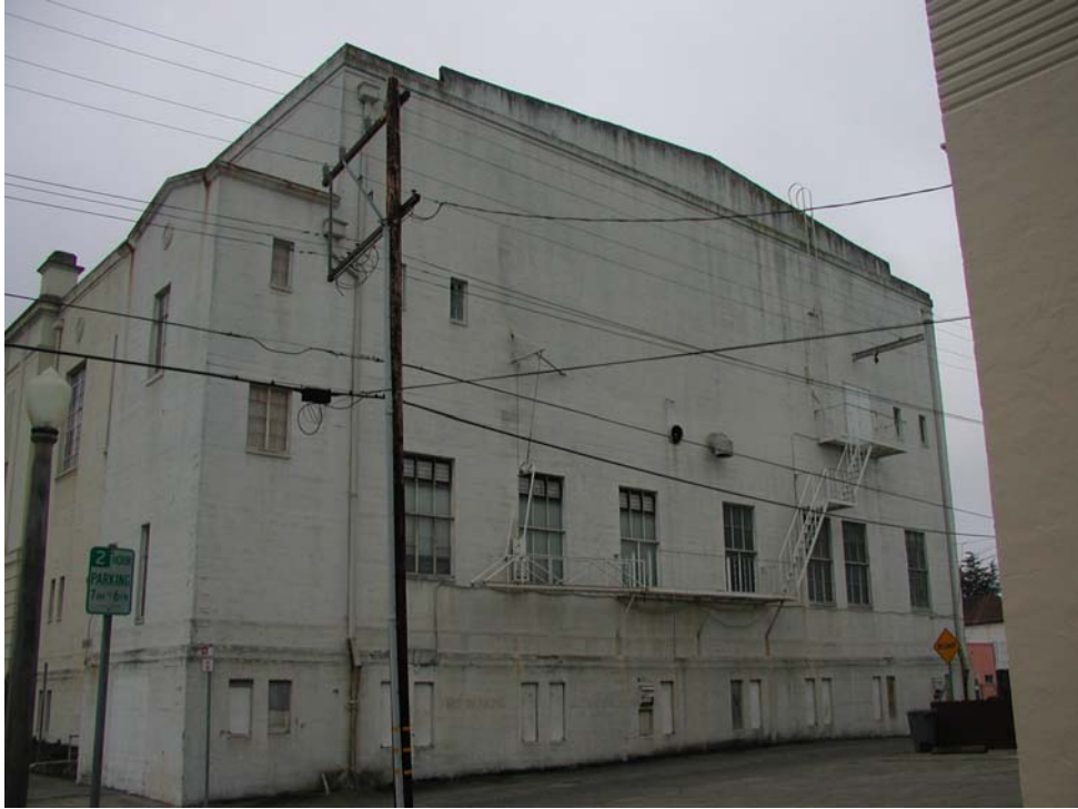
North Elevation – Back of Building (March 2008)
