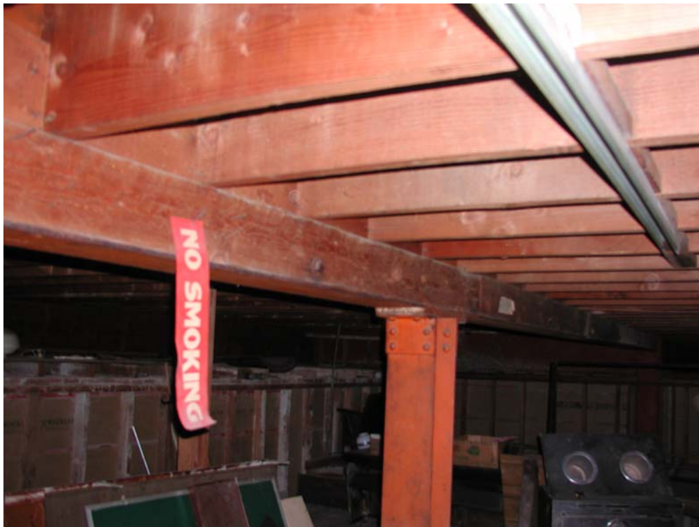
Typical floor framing (March 2008)
