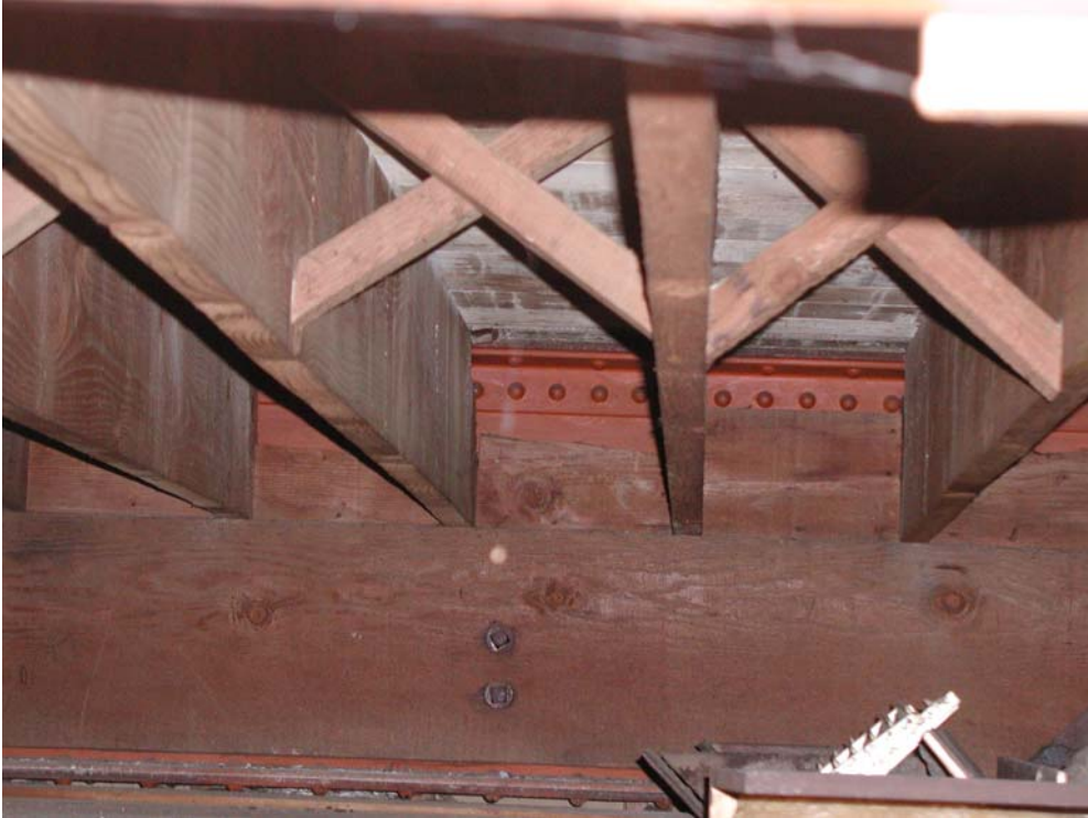
Typical floor framing and steel beam
