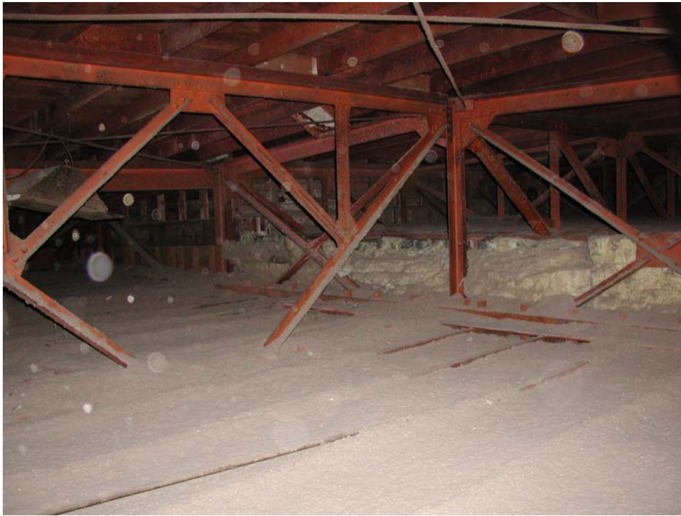
Roof trusses, wood rafters, straight sheathing and ceiling joists
