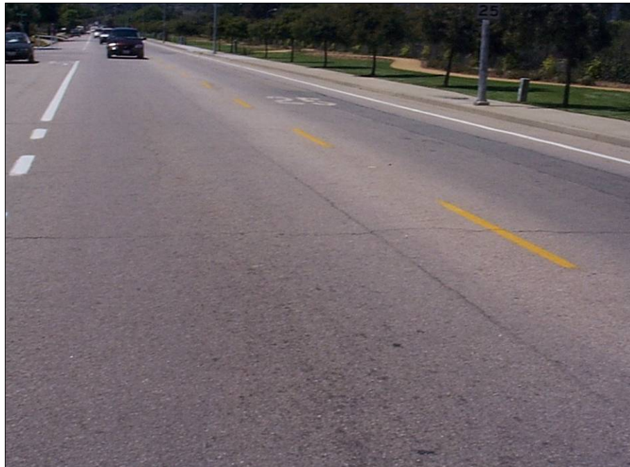
Figure 3.4 PCI = 82 (Good Condition)
